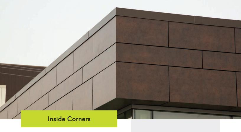
Butt corner pieces are best to be constructed with sintered ceramic slabs 1/4" (6mm) or thicker.
