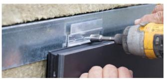
The aluminum clip is attached to the sub-framing using a self-drilling hex screw with an extended hex head driver.
