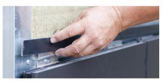
10 **Horizontal** infill strips are then installed across the top of the row of panels.
