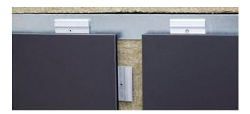
7 Repeat steps 3-5. The next panel is placed onto the J-trim and slid over to connect with the previous panel installed.
