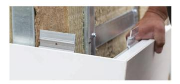
Mitered corners or jambs are installed in the same manner flat panels are installed.
