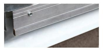
1 J-trim is mounted to the sub-framing at the base of the wall over top of the flashing.
