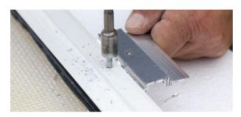
The panel is placed face down on a table and the aluminum clips are installed to align with the sub-framing system.
