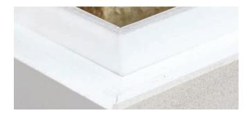
Infill strips can be routered from the back and bent to create a clean corner.
