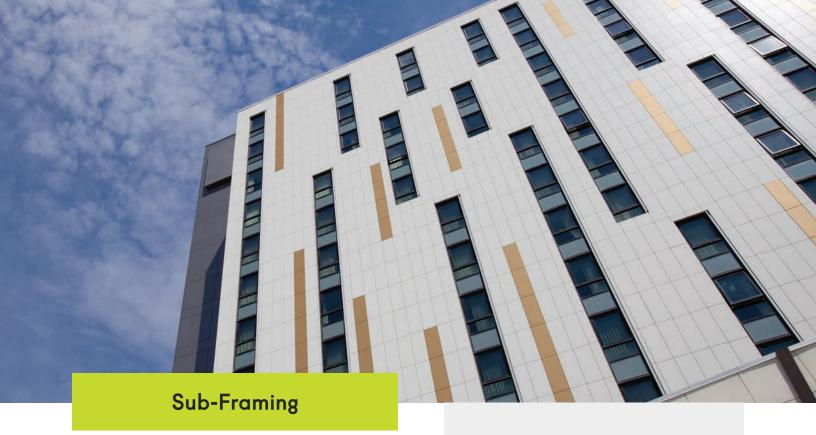
The Ceramitex® Sintered Ceramic Facade System can be mounted on a vertical or horizontal adjustable thermally broken galvanized framing system. Framing can be installed vertically or horizontally on concrete block or poured concrete but in most cases vertical framing is used. If the substrate is constructed with vertical steel studs, horizontal framing is preferred. The project design will dictate how the sub-framing will be installed.
