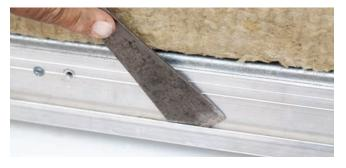
2 Before installing the panels, the installer must ensure that the J-trim is clear of all debris.
